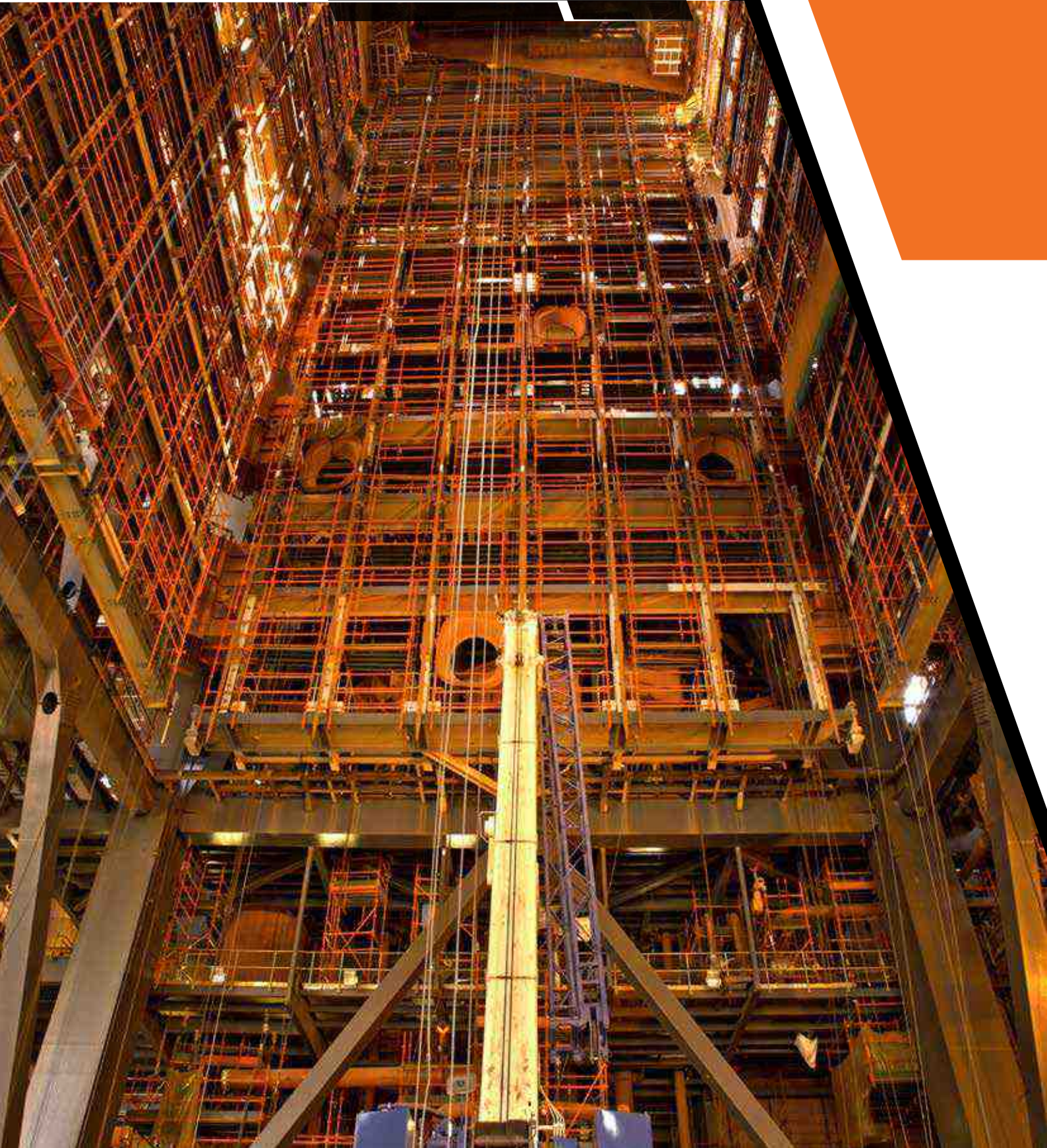
Kusile Power Station, 2015
